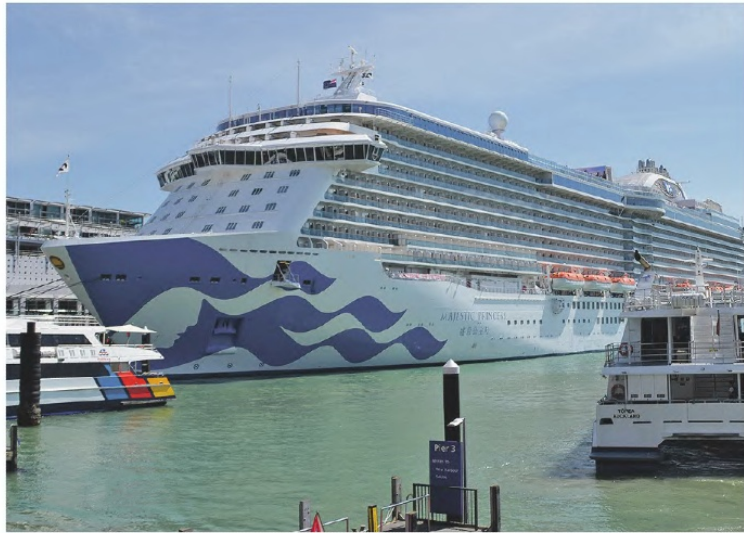
The proposed works include the construction of two new ship mooring dolphins each supported by six 1.8m-diameter concrete piles to enable large cruise ships to berth. Photo Sophie Boladeras
